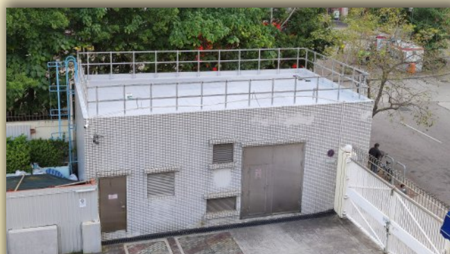
New facility Fencing for the switch room rooftop
